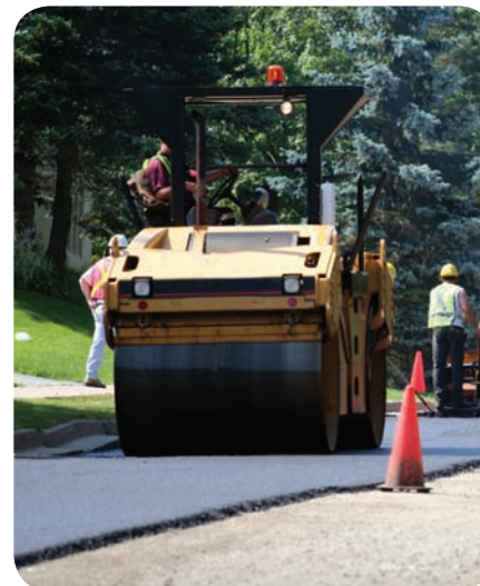
▲ The new road surface is bitumen mixed with fine gravel.
