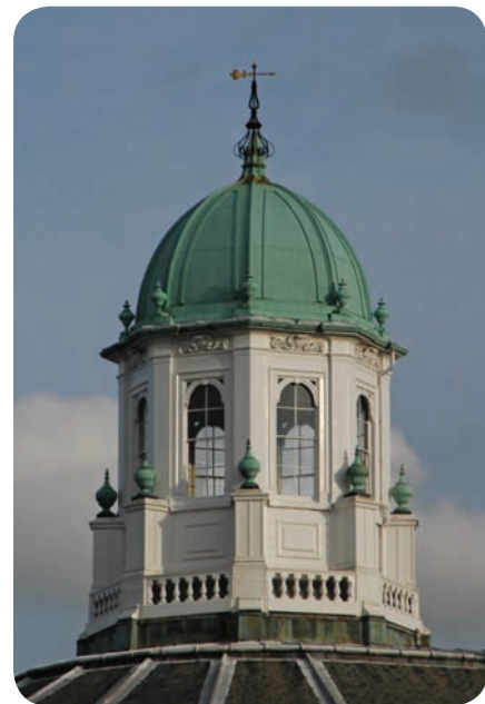
▲ Copper is used for roofing, since it is unreactive. But over time it does form a coat of blue-green copper(II) carbonate.
