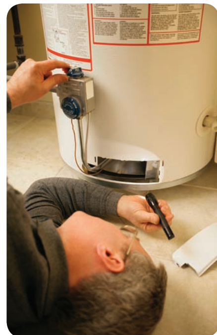
▲ Gas-fuelled water heaters and boilers should be checked regularly. Every year, hundreds of people are killed by carbon monoxide from faulty burners.
